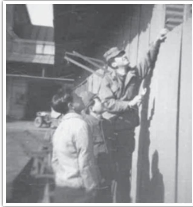
Carl and his Japanese assistants working on an electrical problem in the factory.
